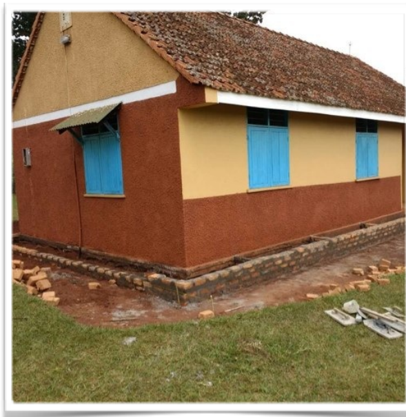
Left: masonry work in progress outside the HIV Clinic.
